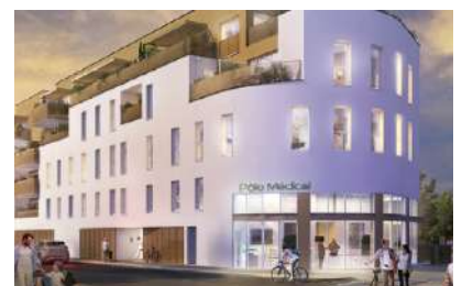
Villenave-d'Ornon (33) MedCorner City (cabinet médical)
